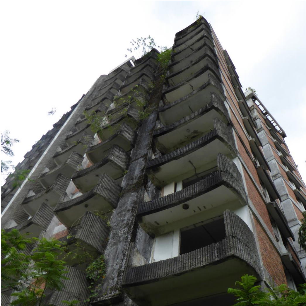
Highland Towers, Malaysia © Veronika Fendel
