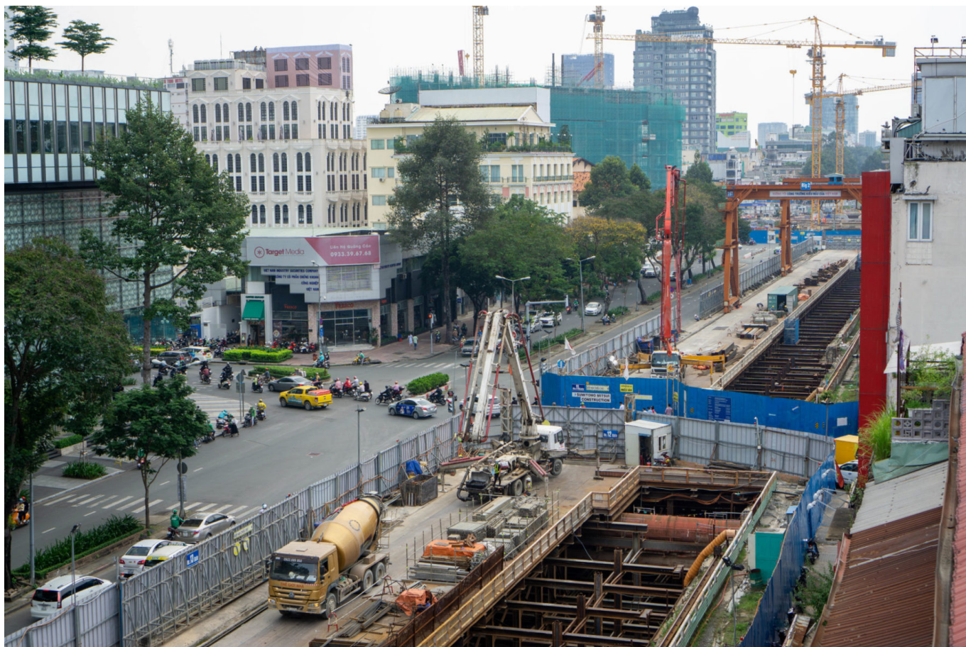
Bau der Metro in Ho Chi Minh City © Marco Verch, Flickr, CC BY 2.0
